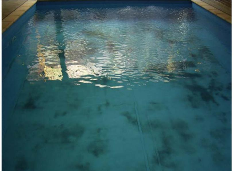
At first sight the solution seems simple : avoid the presence of bacteria behind the membrane or avoid the presence of metals in the swimming pool water; in both cases this would eliminate the formation of metal sulphides. In practice however, it is quite difficult to remove completely all bacterial activity behind the membrane. Nor is it possible to avoid the presence of a low quantity of metals salts in the swimming pool water.
